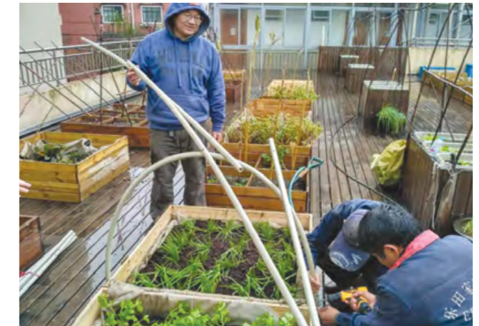
Installing raised bed boxes on the rooftop of Shixi Primary School
